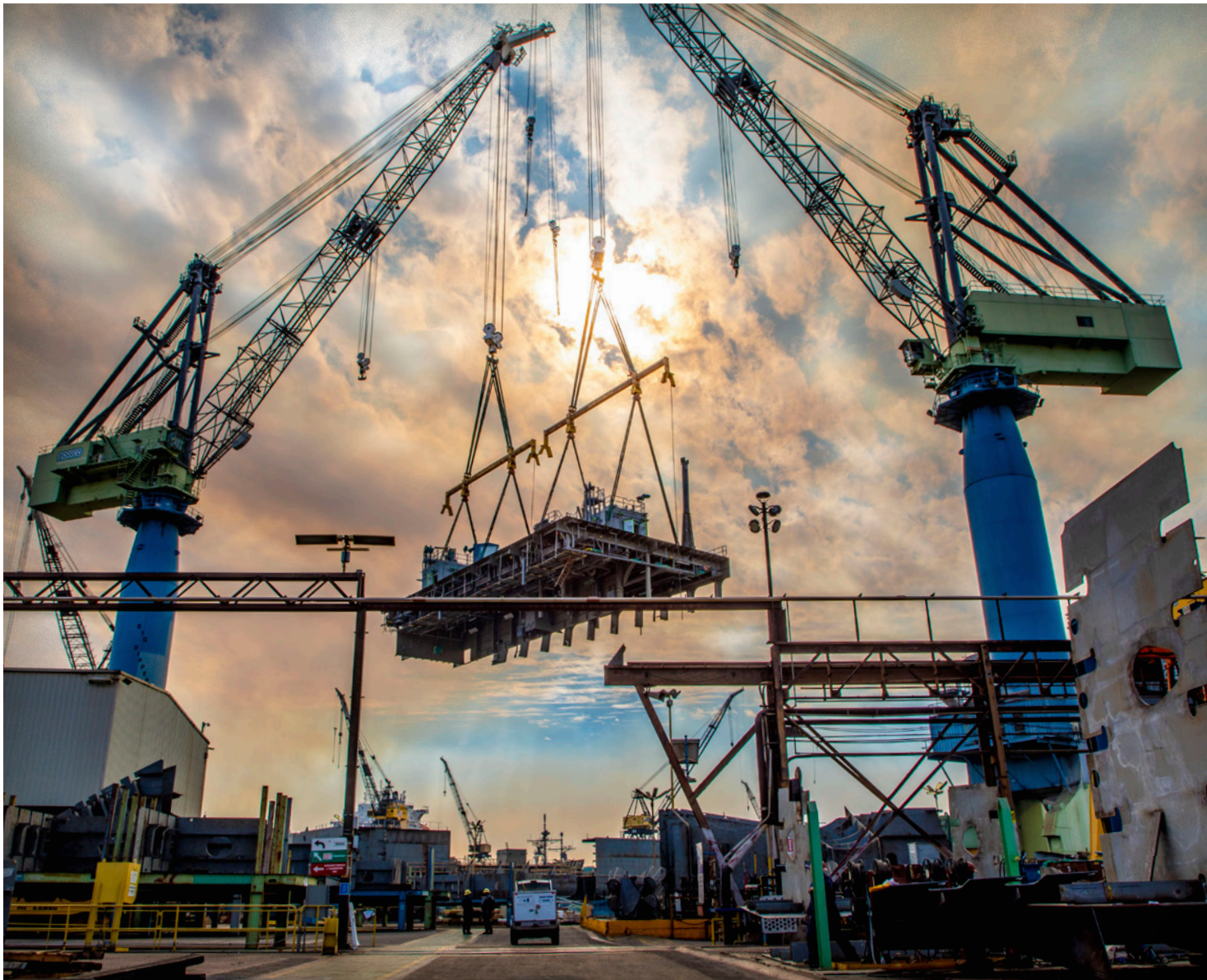
John Lewis-class fleet replenishment oiler construction at NASSCO
